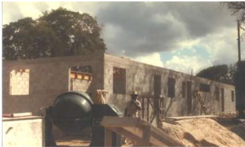
Female Ward under construction.
