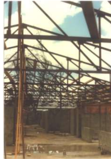
Pediatric ward-Phase 1 wing under construction - view down main corridor.
