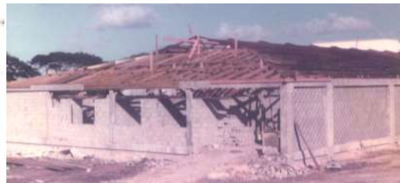
Pediatric Ward Phase 1 roof framing.
