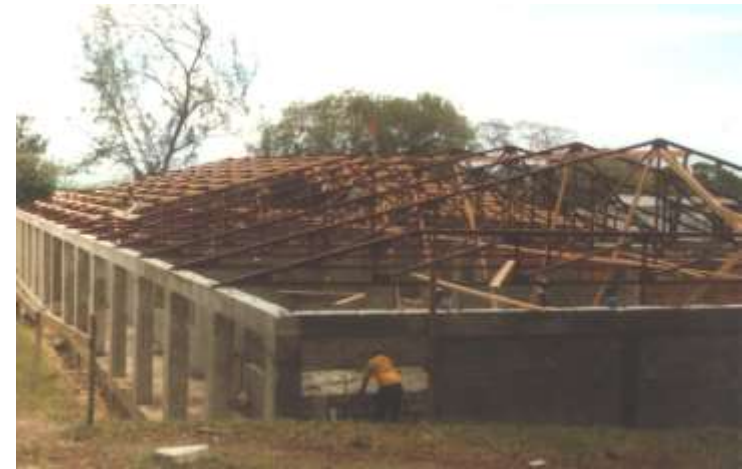
Pediatric Ward-Phase 1 under construction.
