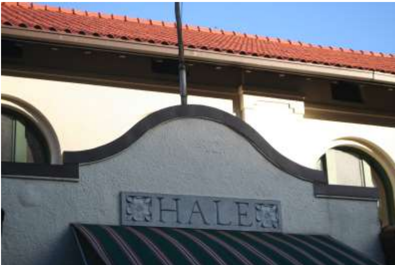
Exterior sign detail.
