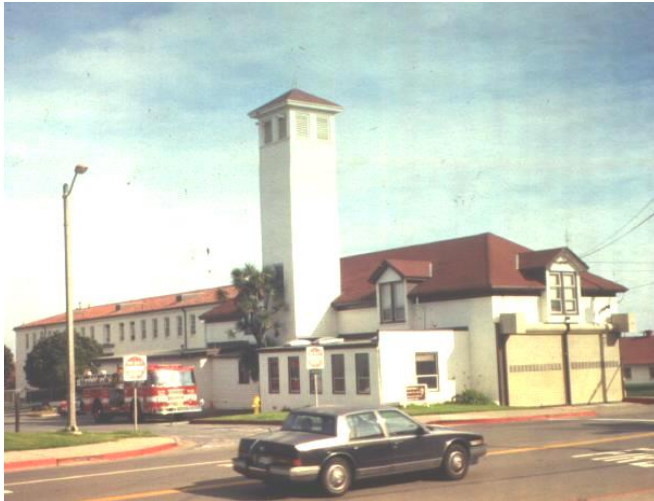
Presidio Fire Station before rehabilitation.
