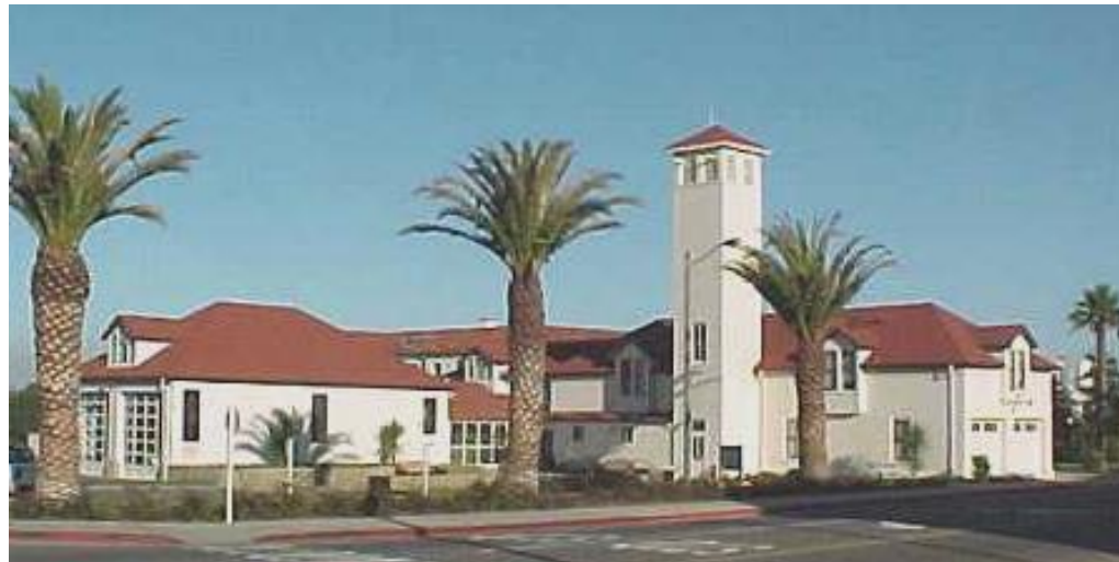
Rehabilitated fire station with the new apparatus bay wing at left.
